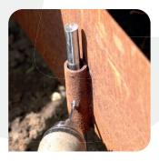
Once the edging is in place, adjust the height by sliding the edging up or down on the pins. This allows you to create your datum, ensuring the edging is level and at the correct height. Once the desired height is achieved, lock it in place using the DatumLock<sup>TM</sup> screws.
