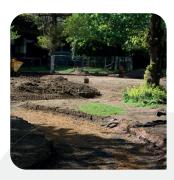
Begin by clearing the site thoroughly and preparing the sub-base as necessary to ensure a stable foundation for the edging.
